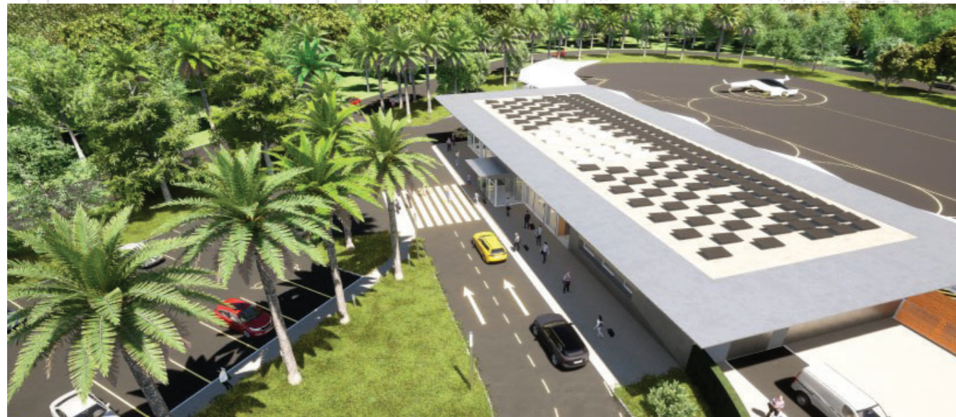
AECOM and Ferrovial have partnered to design a network of vertiports connecting strategic locations in major Florida cities
